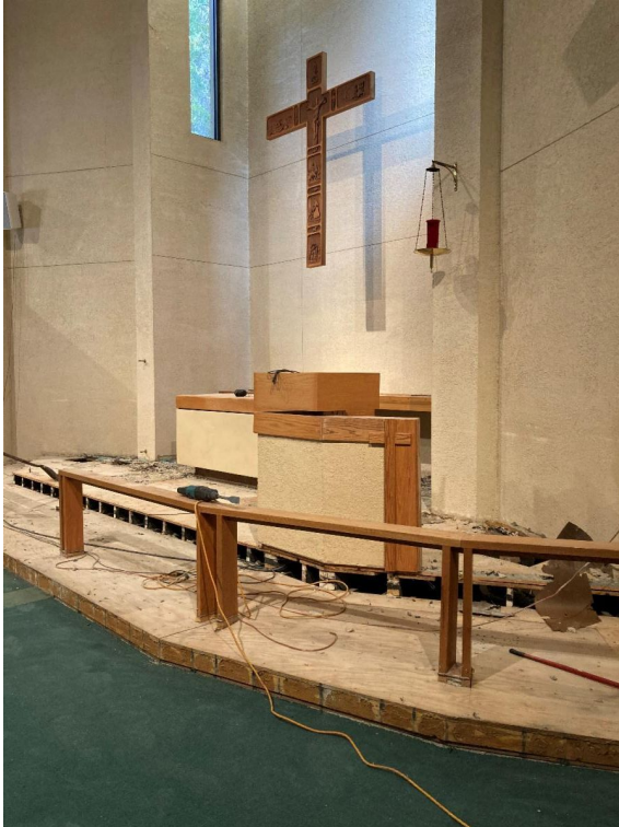
Old flooring and ventilation ducts being removed and readied.
